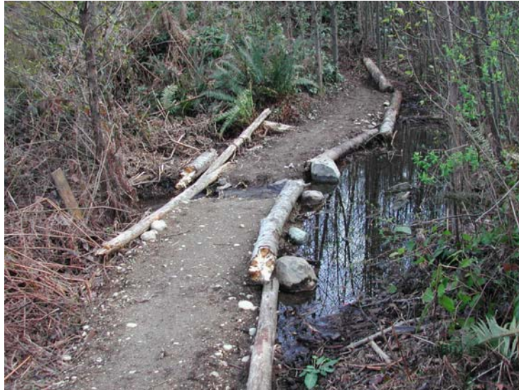
Section III trail blocks stream flow
