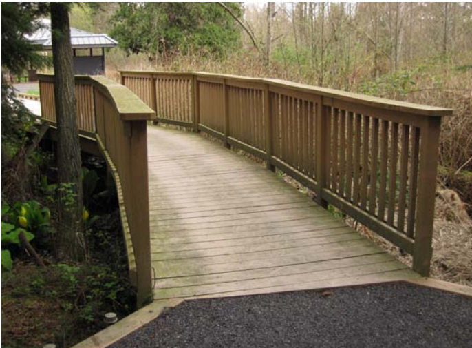
The boardwalk crossing at Rotary Community Park in Woodinville.
